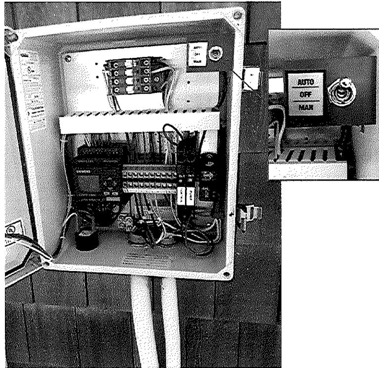
Usually it's the high water alarm that sounds. After silencing the alarm, open the control box. Locate the toggle switch on the upper right side. Flip the switch to "Manual". The pump will come on. The pump moves about 10 gallons of effluent out of the tank every minute. Run the pump for about 5 minutes, then switch it back to "Auto". The water level should be low enough so that the alarm is not reactivated in 12 hours.
