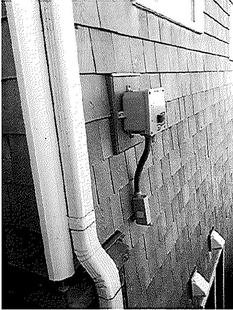
A septic alarm panel is located on the side of each unit. If there is an alarm, the lighted button glows. To silence the alarm, push the button. There is also a PUSH TO SILENCE button on the main septic control panel at the back of the house.
